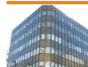
4 Livecon Engineering Co., Ltd Head office/ 1-8-8 Kajicho, Chiyoda-ku, Tokyo 101-0044
