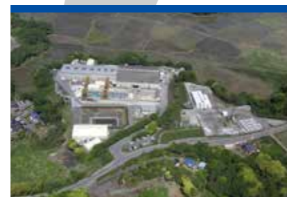
1 Ibaraki Dai-ni Work Location 2744-3, Aso, Namegata, Ibaraki Prefecture 311-3832 Site Area TEL: +81-299-72-3336 Building Area 51,600m 2 Stockyard 6,000m 2 129,300m 2 (Shared by Ibaraki Dai-ichi Plant / Ibaraki Dai-ni Plant)
