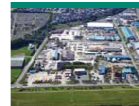
6 AIZAWA Concrete Corporation Plant/ 2-2 Koeicho, Ebetsu, Hokkaido Prefecture 067-0051
