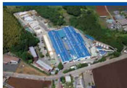
1 Ibaraki Dai-ichi Work Location 3347-1, Aso, Namegata, Ibaraki Prefecture 311-3832 Site Area TEL: +81-299-72-0851 Building Area 53,500m 2 (including yard) Stockyard 9,000m 2 129,300m 2 (Shared by Ibaraki Dai-ichi Plant / Ibaraki Dai-ni Plant)
